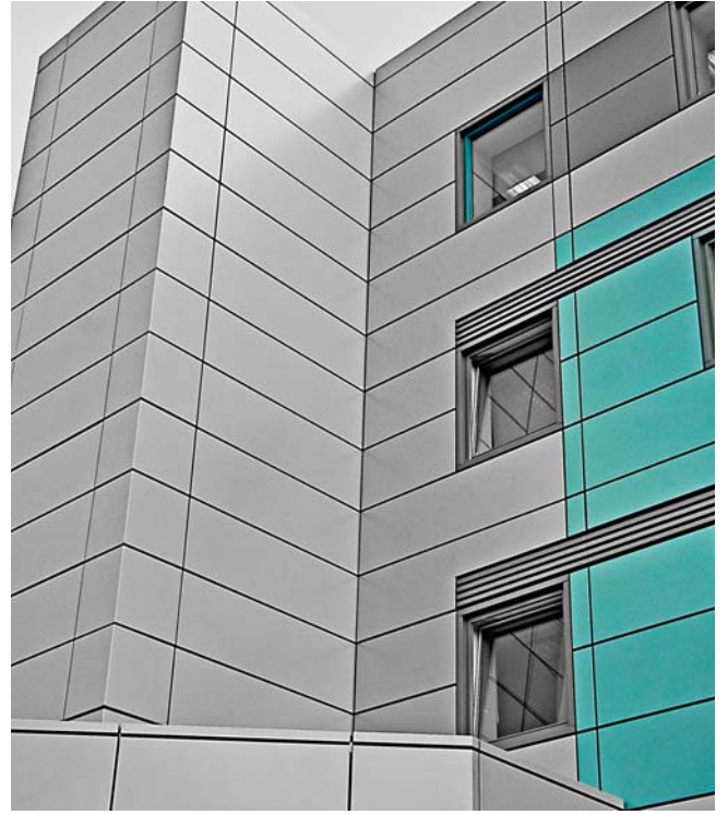
Bedford College, Workshop Building after
