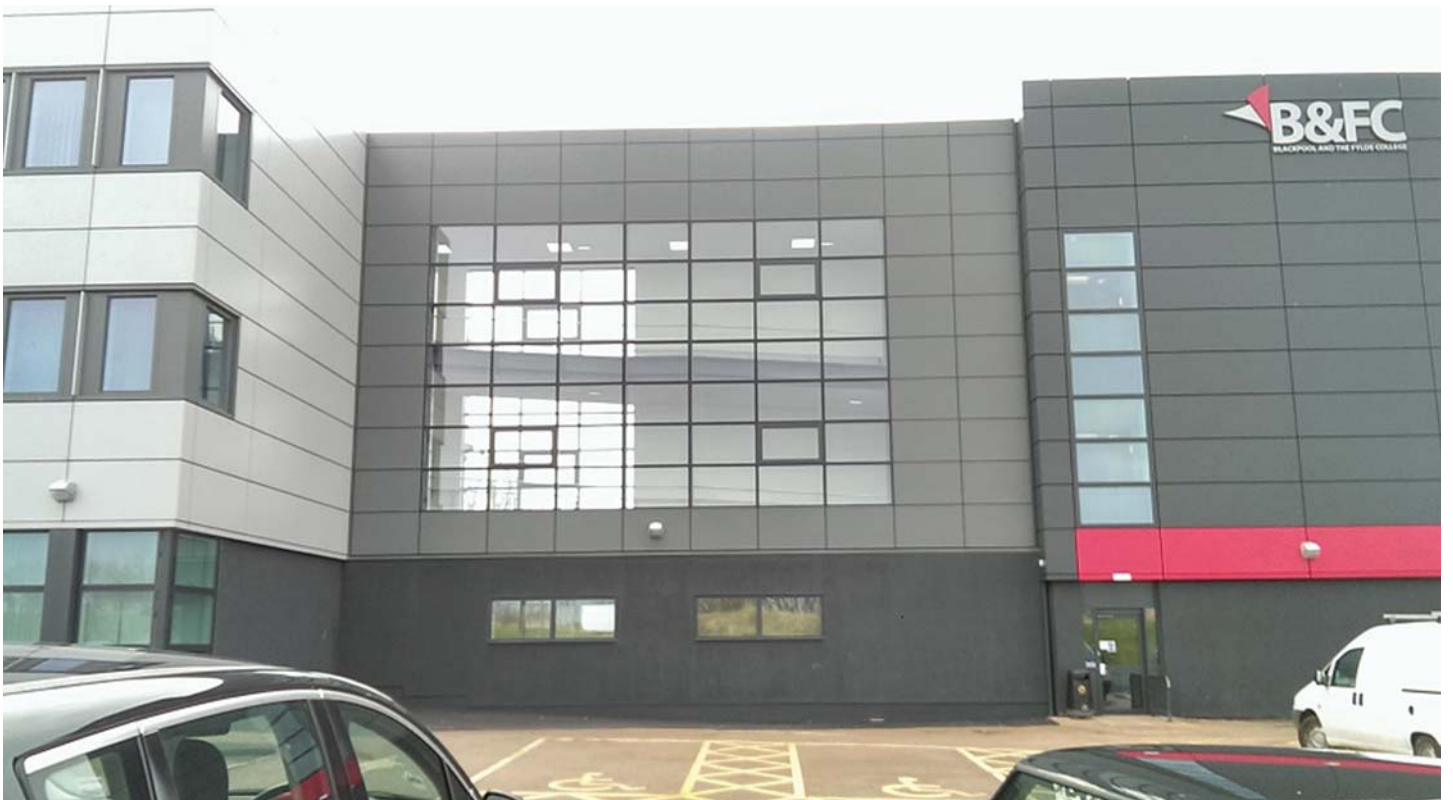
New-build Thornton Elswick link enhancing accessibility between buildings
