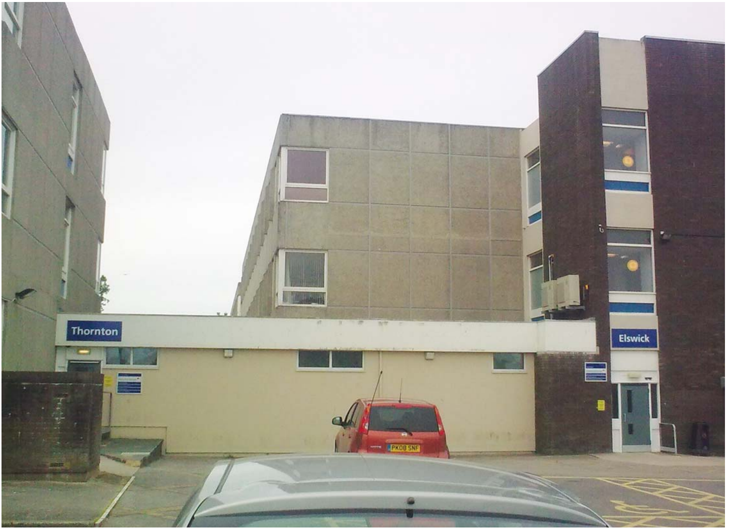
Existing Thornton Elswick low-level link
