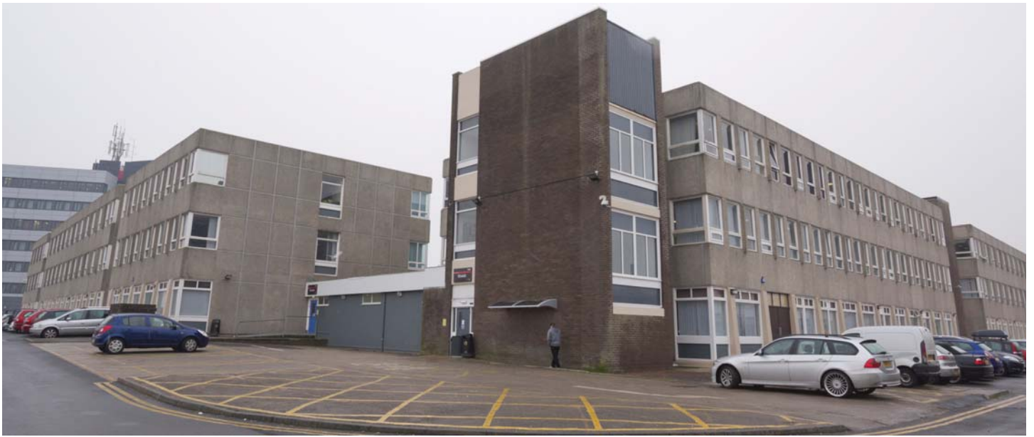
Cleveys building completed as Phase I in 2012 can be seen in the background with Phase II in the foreground
