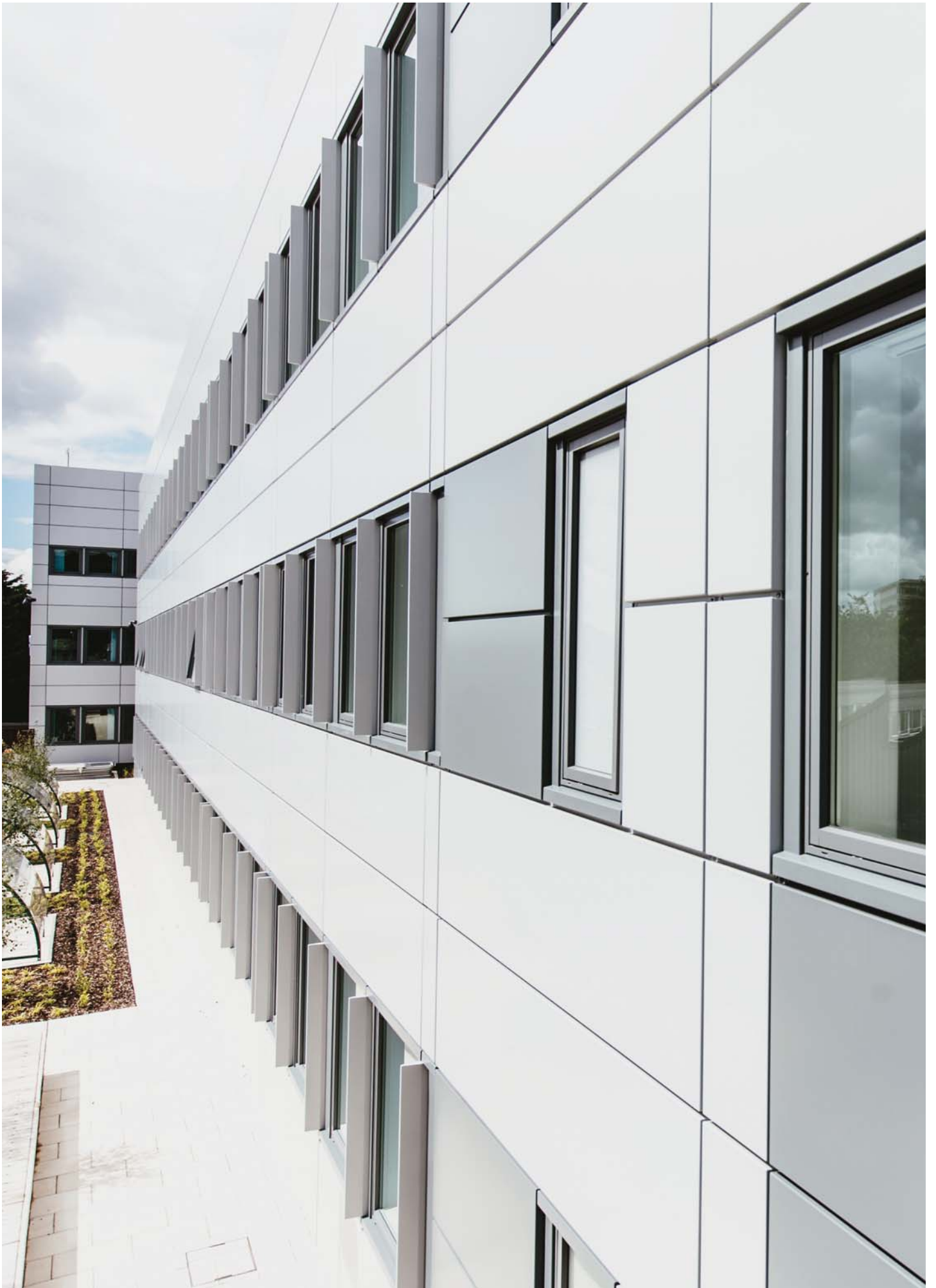
The Bournemouth & Poole College, Applied Science and Digital Media Building
