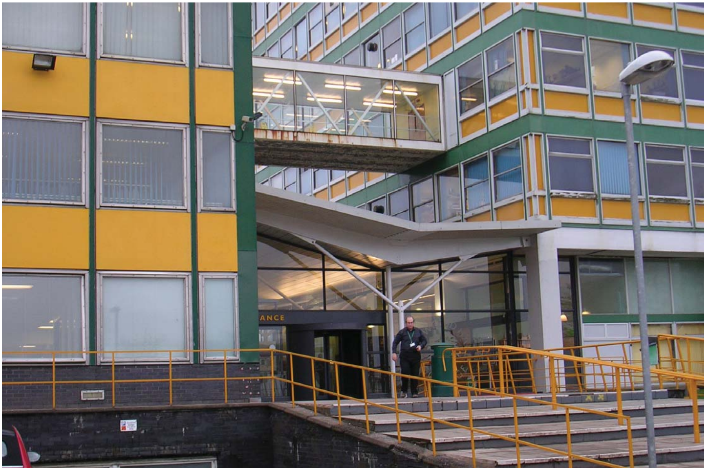
Hopwood Hall College, Rochdale before
