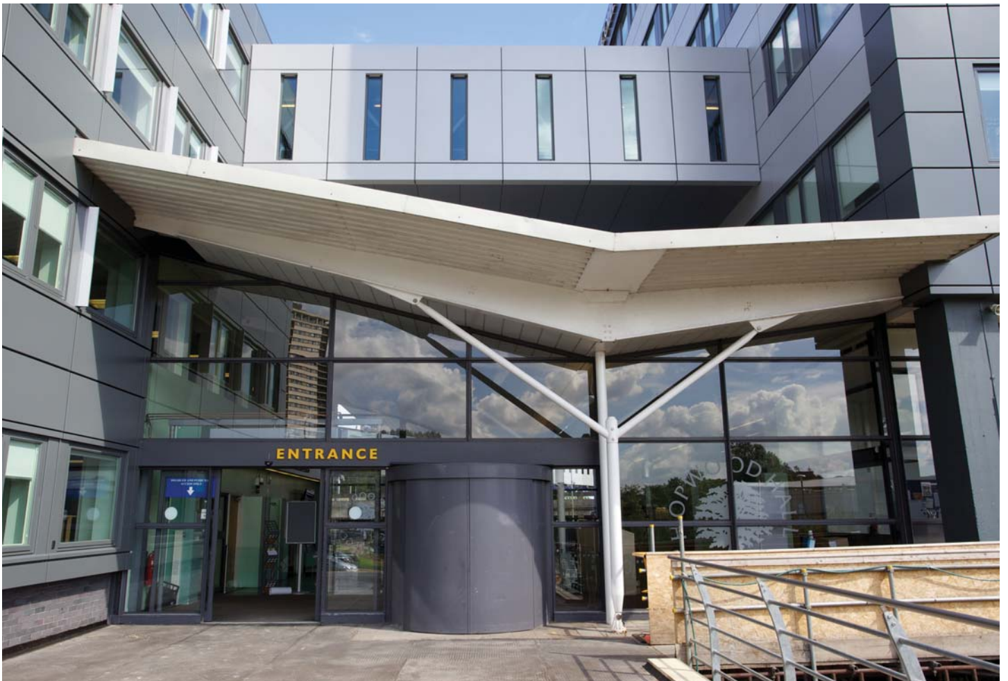
Hopwood Hall College, Rochdale after
