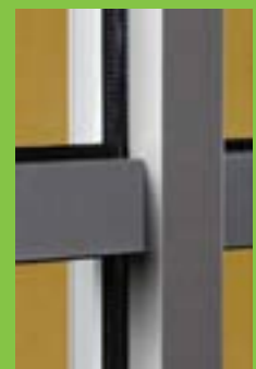
Curtain Walling Total wall construction mainly of double-glazed units supported on an aluminium framework.
