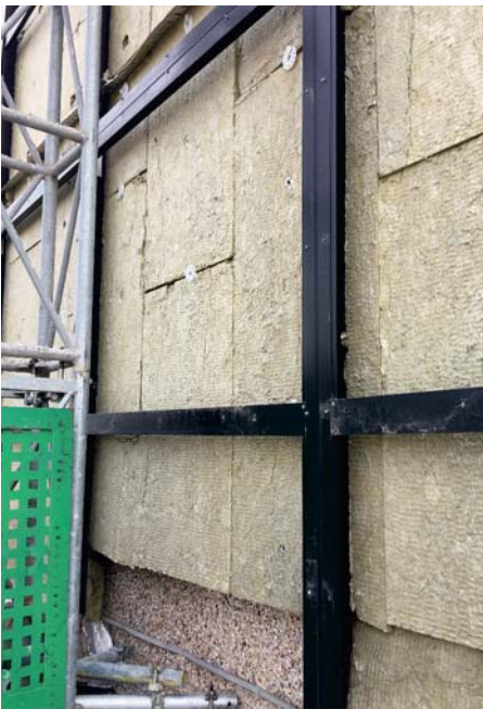
Insufficient fixings in insulation.
