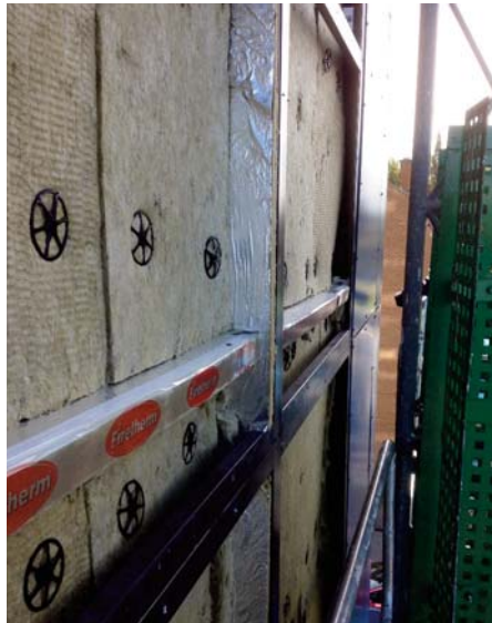
Closeup of new firebreak & insulation.
