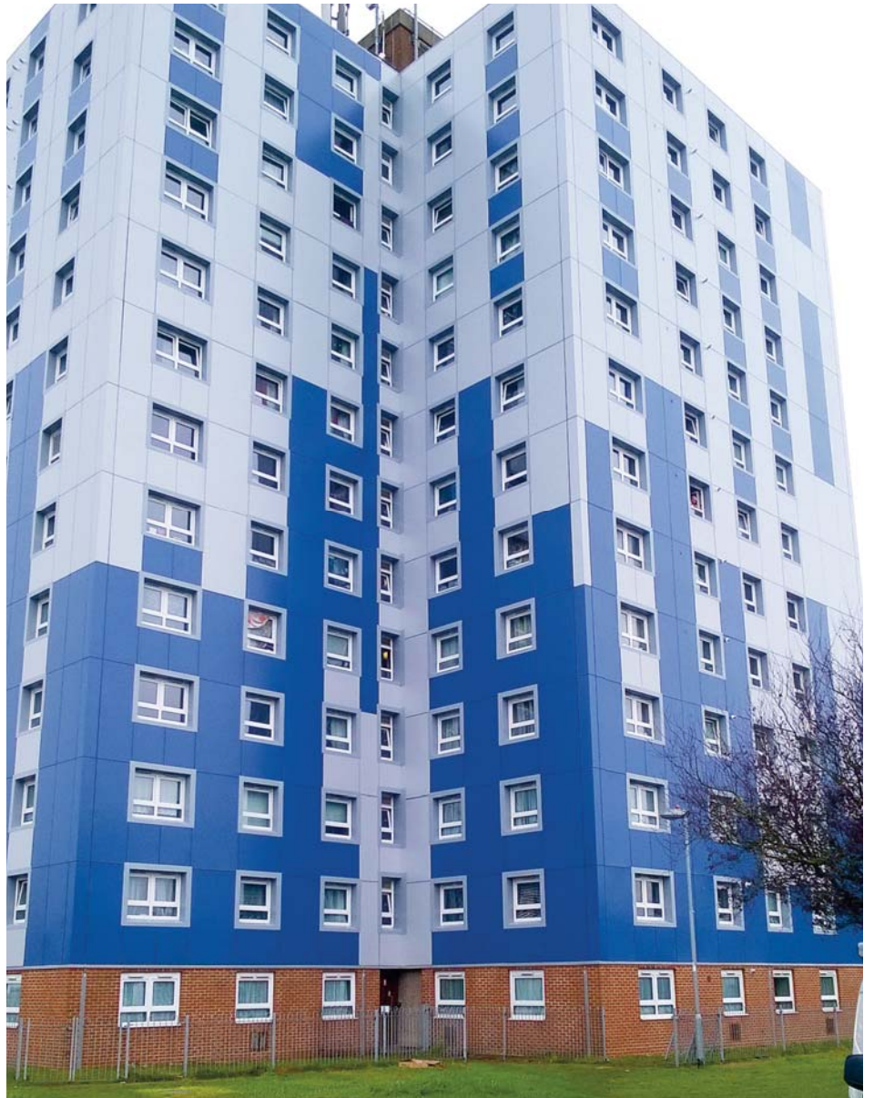
Non combustibile cladding complete to surpass current standards.
