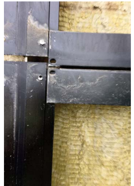
Missing support structure fixings.
