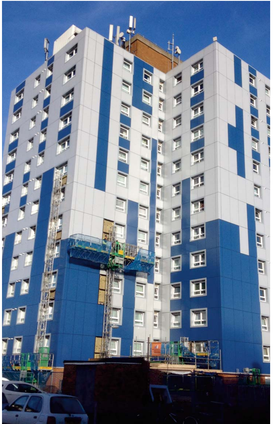
Access under removal.
