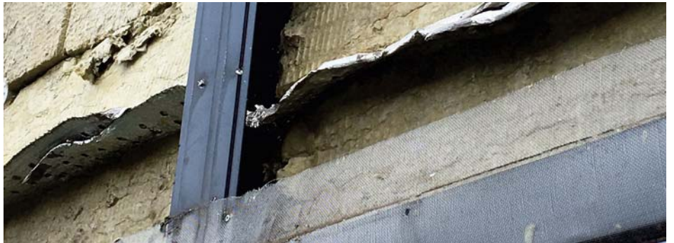
Incorrectly installed firebreaks.
