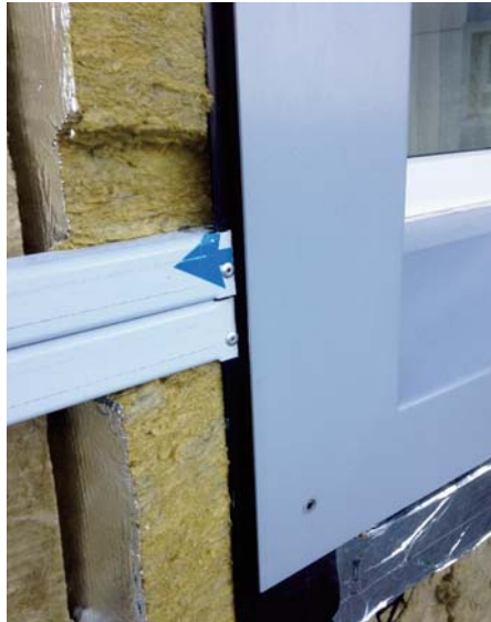
Support structure replaced where missing.
