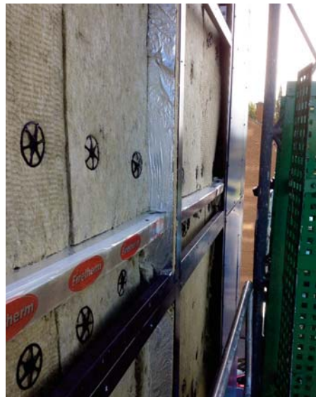
Closeup of new firebreak & insulation.
