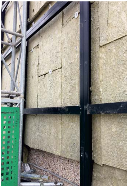
Insufficient fixings in insulation.
