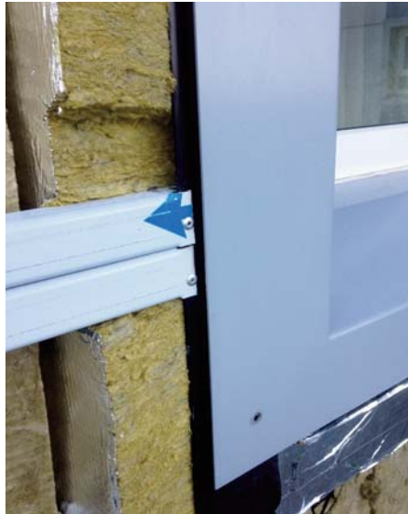
Support structure replaced where missing.
