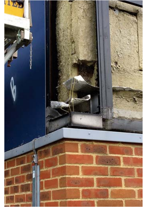
Incorrectly installed firebreaks and gaps in insulation.
