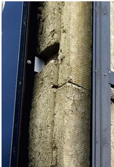
Gaps in insulation and support structure missing.
