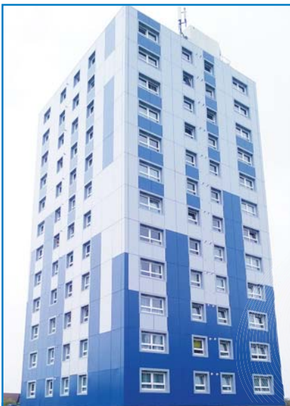
Clements Court 27th October defective overcladding stripped and replaced.
