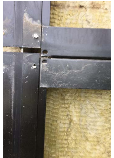
Missing support structure fixings.
