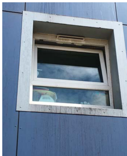
Window and POD before clean and cladding replacement.
