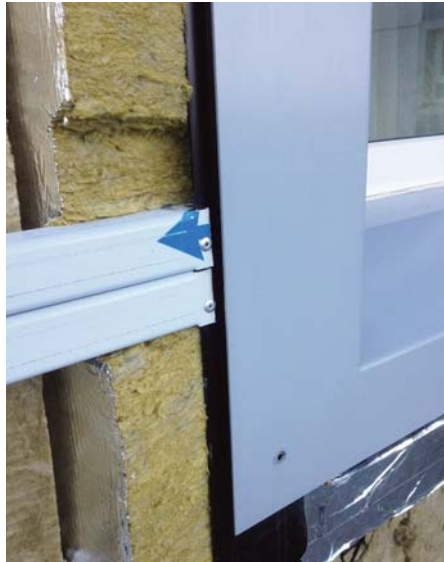
Support structure replaced where missing.
