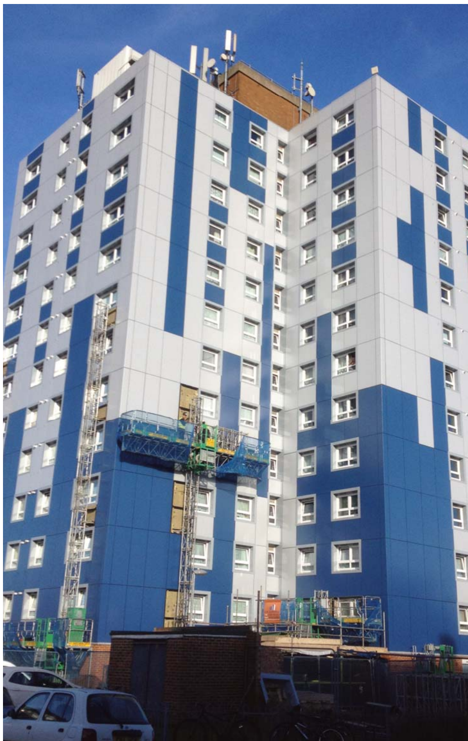
Access under removal.
