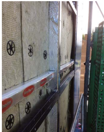
Closeup of new firebreak & insulation.
