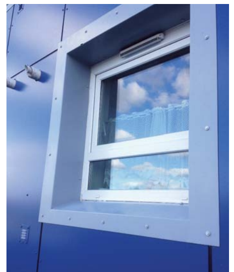
Window and POD clean after new cladding installed.
