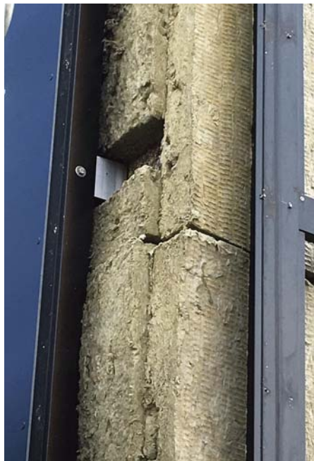
Gaps in insulation and support structure missing.
