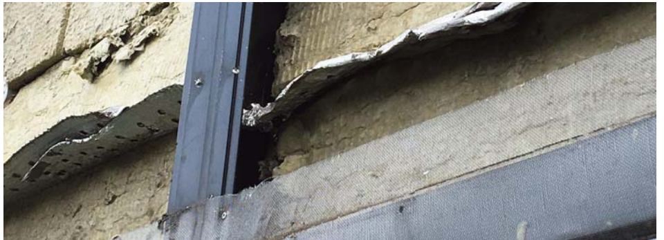
Incorrectly installed firebreaks.
