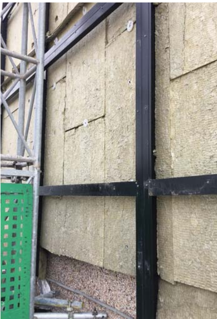
Insufficient fixings in insulation.
