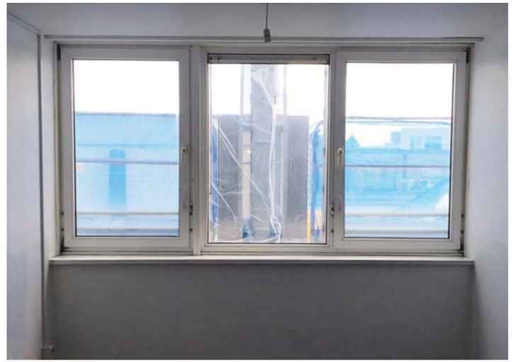
Hockmore Tower Internal After
