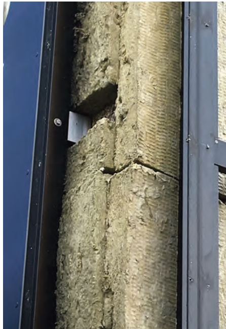
Gaps in insulation and support structure missing.
