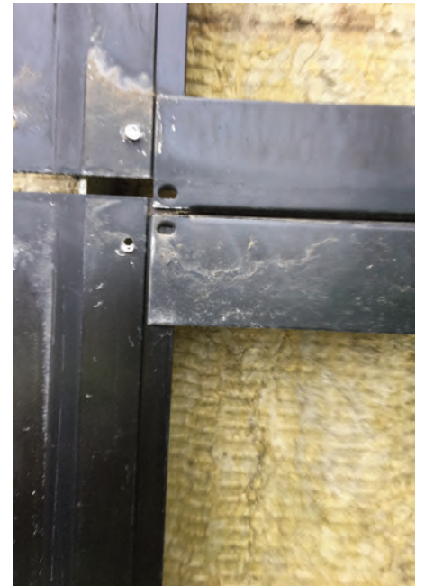
Missing support structure fixings.
