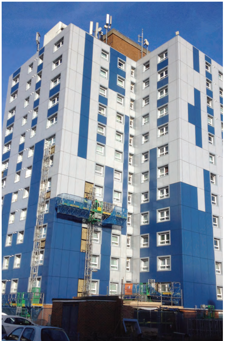
Access under removal.
