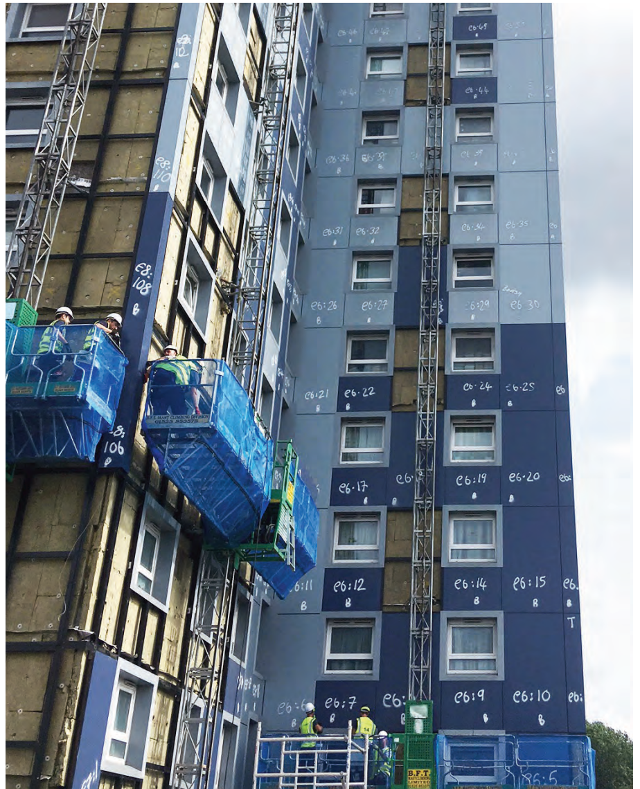
Combustible panel removal.
