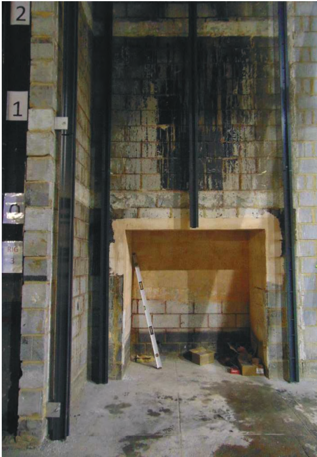
Figure 7. Installation of the aluminium rails up to mid-height.
