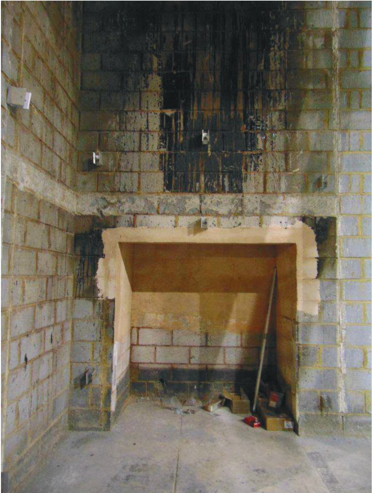
Figure 5. Installation of the aluminium brackets up to mid-height.
