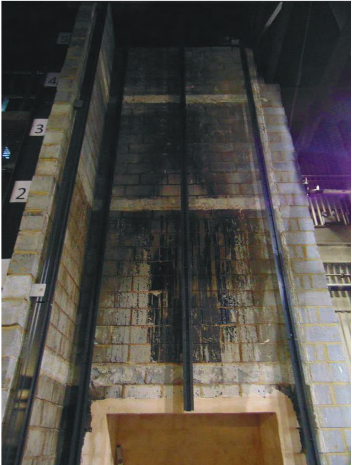
Figure 8. Installation of the aluminium rails up to top of system.
