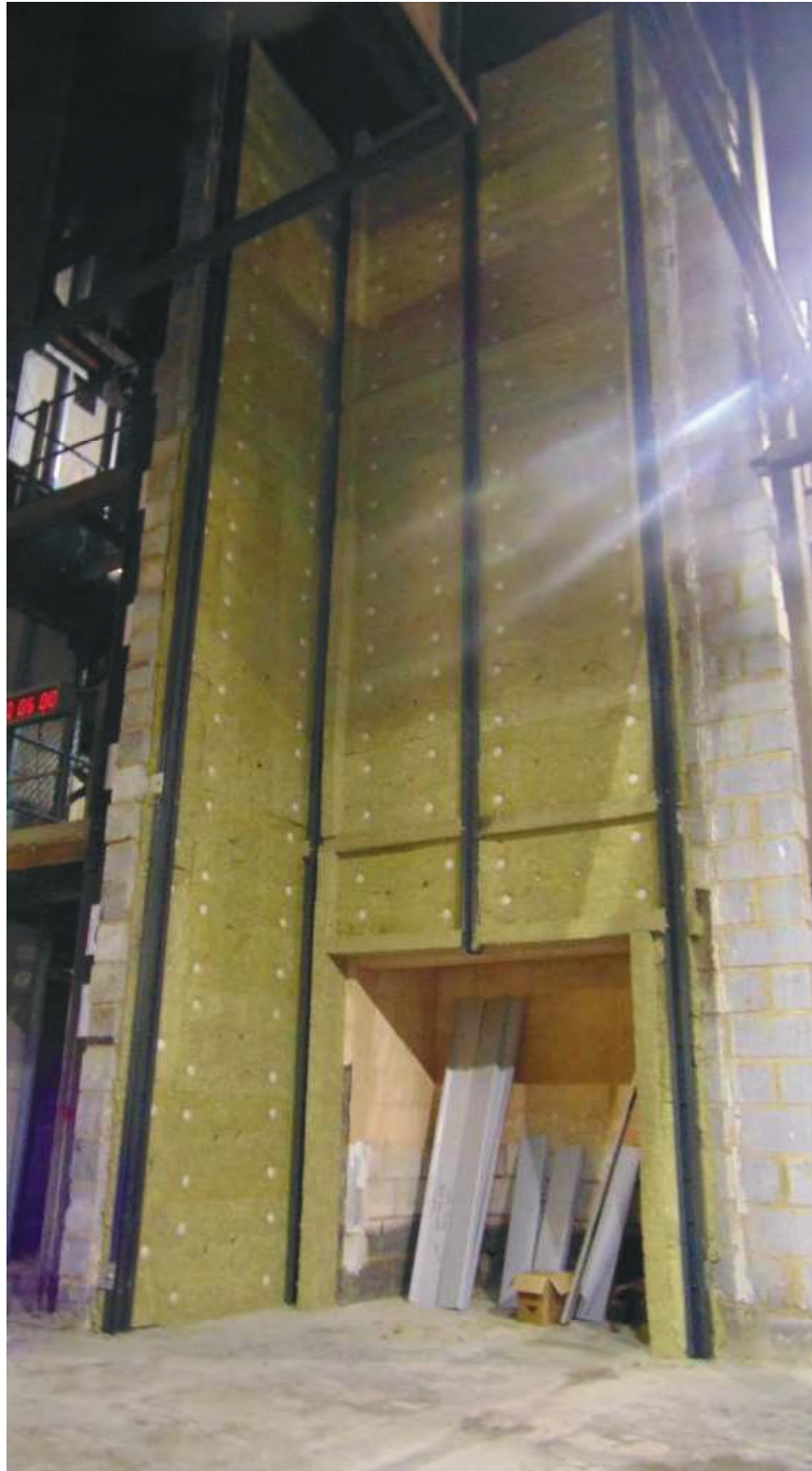
Figure 9. Installation of the insulation, horizontal and vertical cavity barriers.
