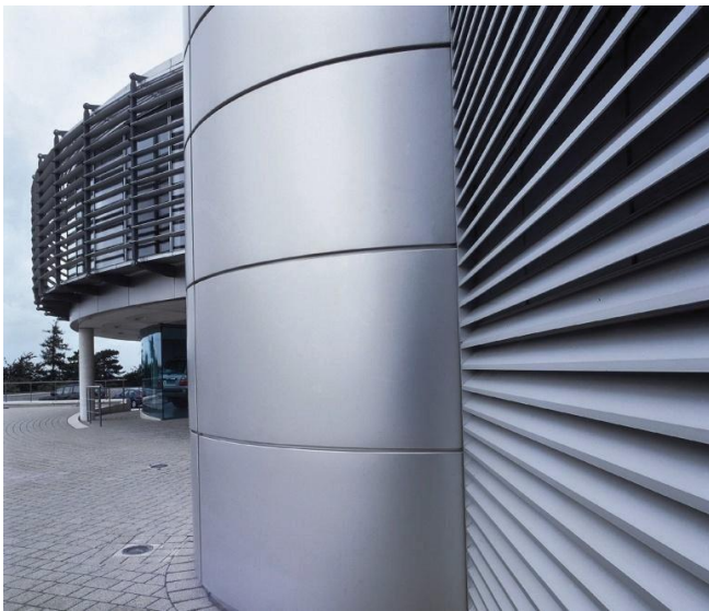
Anodised aluminium can fit different façade forms
