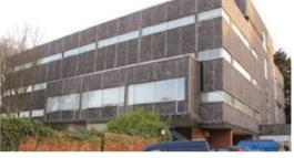
protective scaffolding for some years as its precast aggregate cladding panels have failed and become unsafe. Following a Pre-Contract Services Agreement (PCSA) to assess its structural integrity and determine the scope of works, d+b facades was awarded the contract for aluminium over-cladding, replacement windows, roofing and installation of photovoltaic panels.
