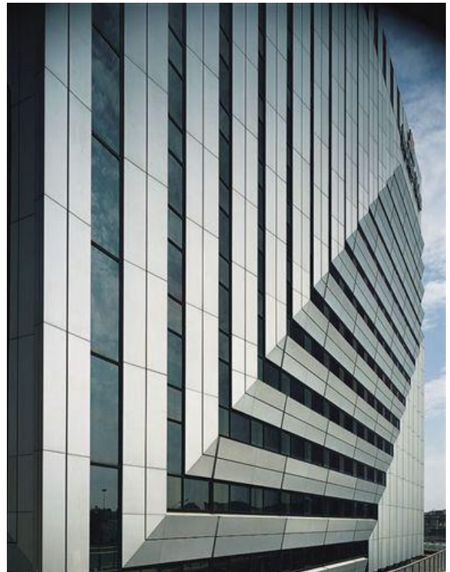
Anodised aluminium can be used to create modern and advanced designs – here on a landmark building in Paris-La-Défense constructed over 25 years ago
